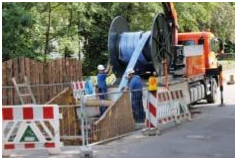
Primus Line being drawn into a pipeline
