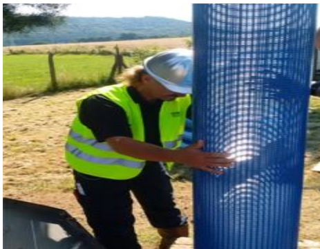
Stainless-steel wire-wrapped screen coated with HAGULIT®
