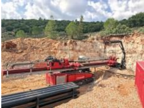
Rock drilling rig
