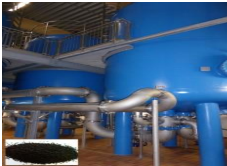
Akdolit® MnFS filter material used in the Hennesee waterworks of Hochsauerlandwasser GmbH
