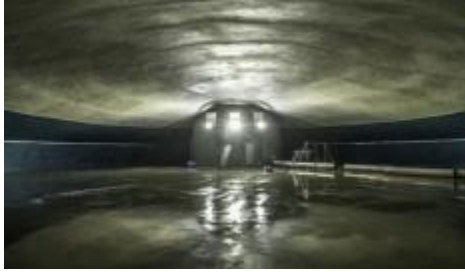
Rehabilitation of tank 2 of the elevated water reservoir in Hewingsen
